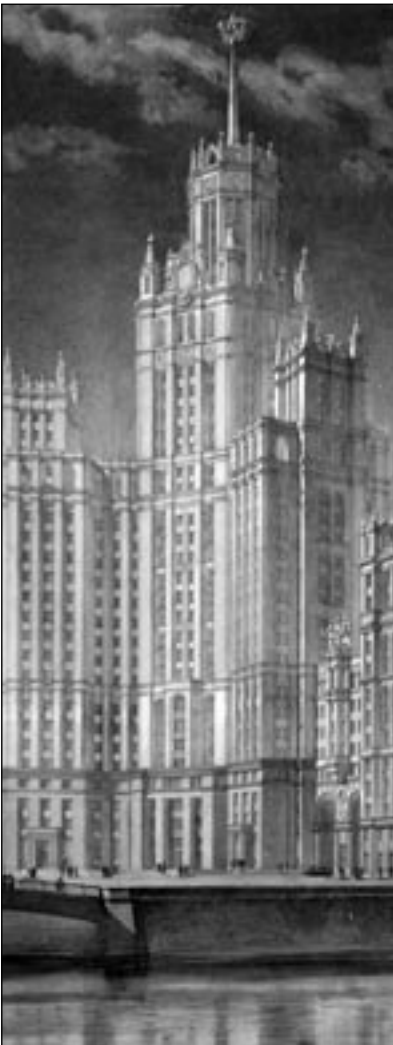
D Chechulin - The administrative building in Zaryadye © Schusev
