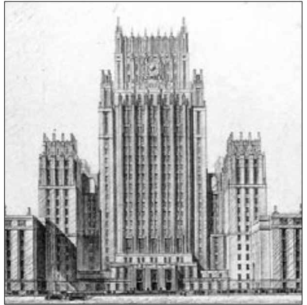
D Chechulin - The administrative building in Zaryadye © Schusev
